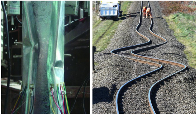
FIG. 1. (Color online) Examples of failure due to compressive stresses. On the left: A steel column that has buckled (in the lab) due to applied compressive stresses (Ref. 6). On the right: a rail track that has buckled due to compressive stress following an earthquake (Ref. 7).
