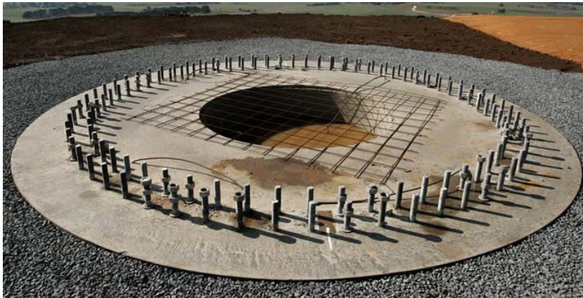
Wind Turbine Foundation ( www.sjwconcrete.com )
